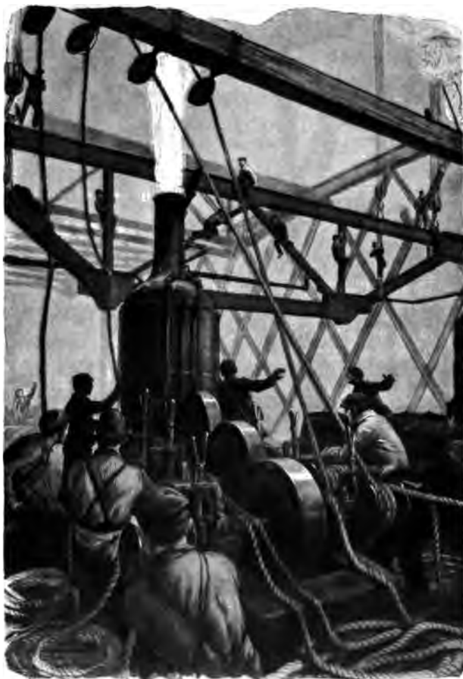
ON THE "TRAVELER." HOISTING A STRUT.
